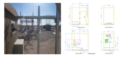
Three key hub sites did not have communication or relay buildings to house the microwave or network equipment. JTS procured and coordinated building installations at these sites. The ground was made ready and communication buildings were lowered into place using a crane.
