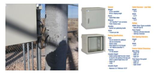
The remote sites at 17 of the sub stations were without any communication shelter. NEMA enclosures were chosen as the most cost effective option to house the equipment connecting back to the hub sites. The NEMA Enclosures were mounted onto 4" poles that were buried 4' into the ground with 6' of the mast exposed. The NEMA enclosure was installed close to the port opening on the concrete pole for the ease of routing the cable to the enclosure.
